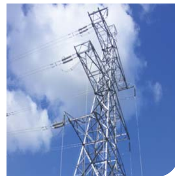
Main image: Second stage build next to live line
